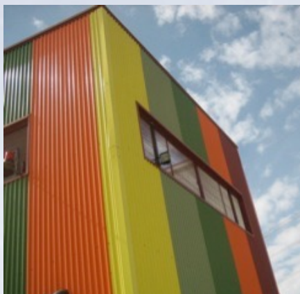
Practicable window open in the reservoir grid
